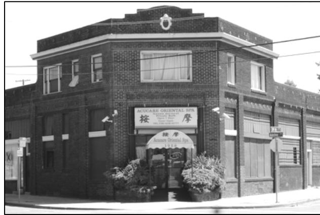
The principal entrance of the building is a two-story office block.
