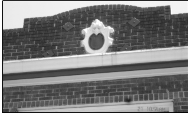
The parapet contains decorative features, including a cartouche that may have contained the Standard Beverages Ltd. insignia.
