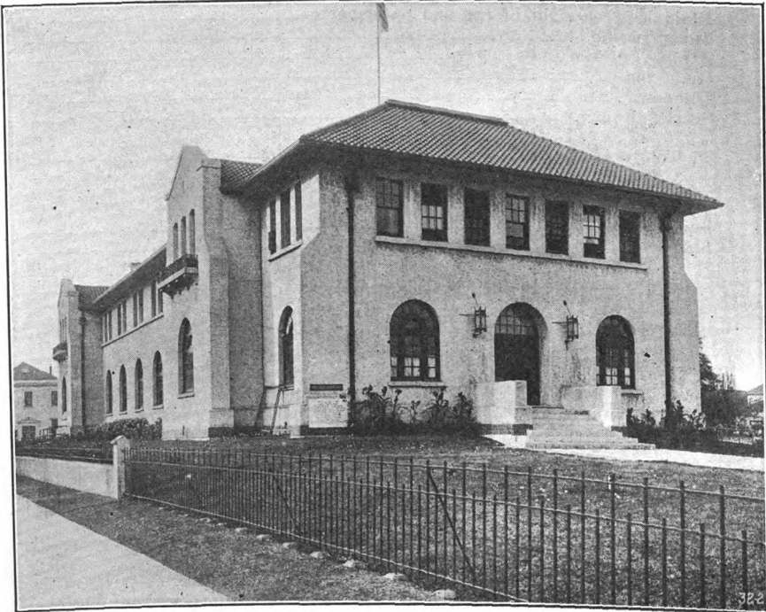
Administration Building, South Side.
